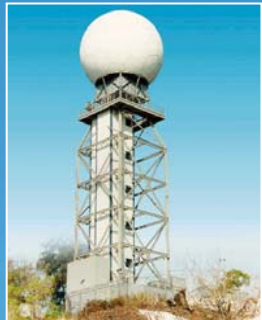
Terminal Doppler Weather Radar (TDWR)
