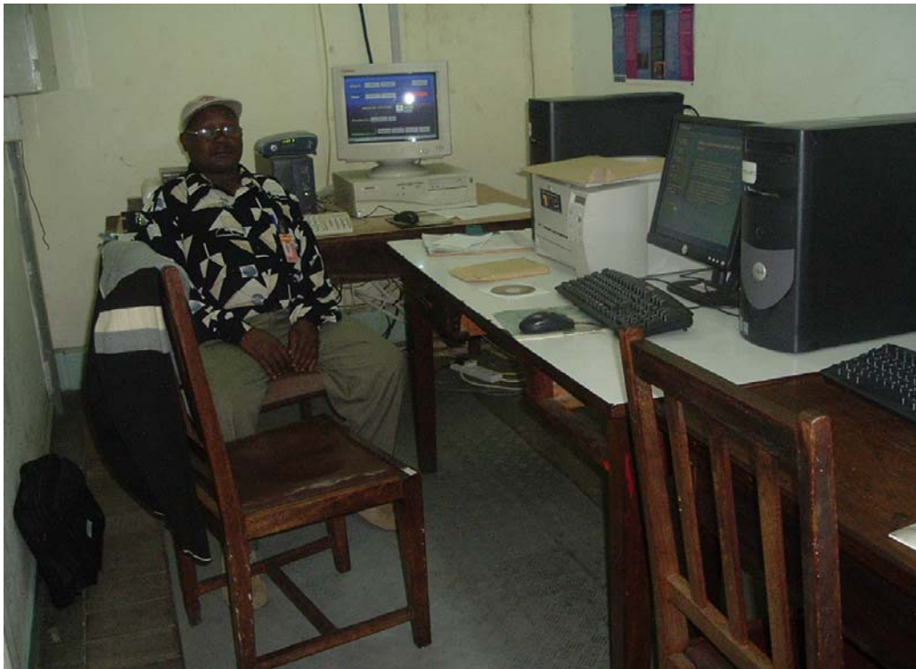
Mombasa MSG and SADIS installation room
