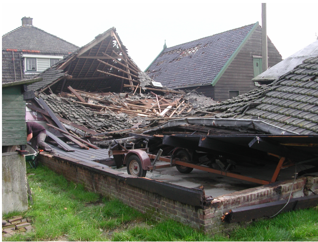
Fig. 5. Damage of a (old) barn due to the tornado in Muiden on 23 August 2004 (photo by R. Sluijter).
