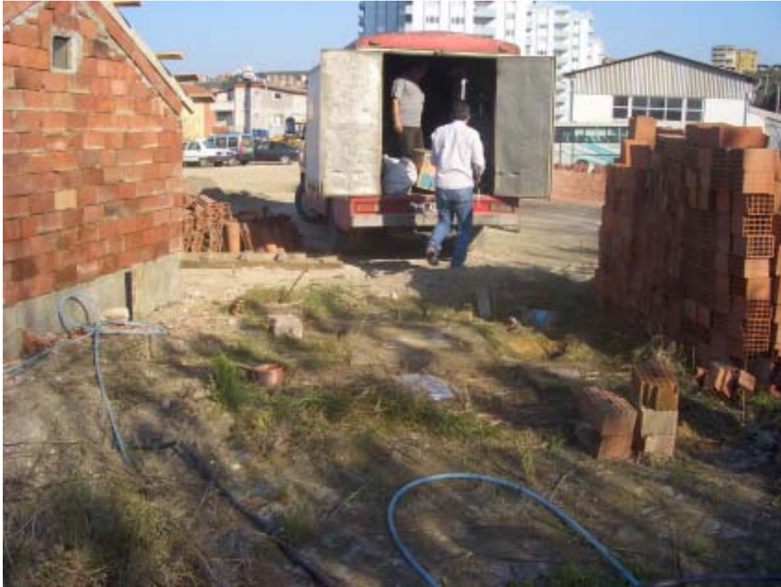
Picture 3: The location for AWOS after pulling up
