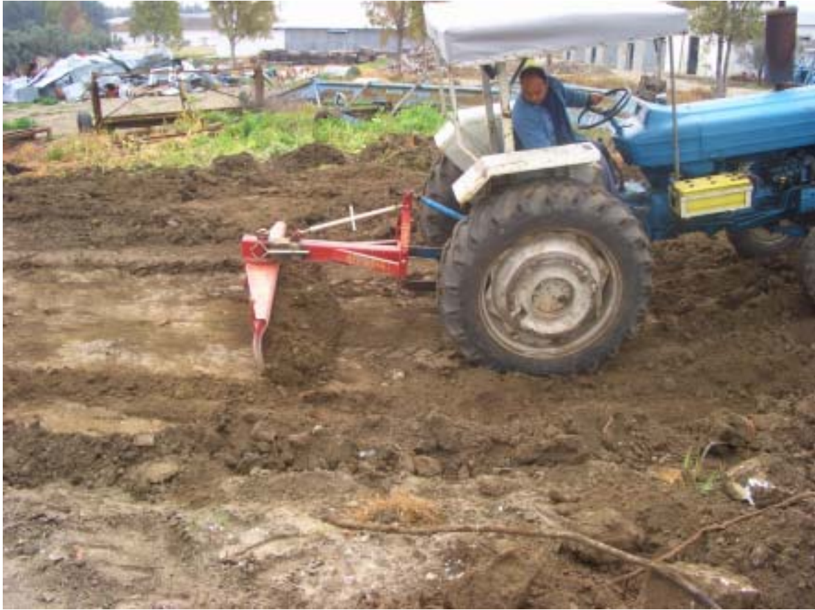
Picture 5: Leveling working for observing park before installation
