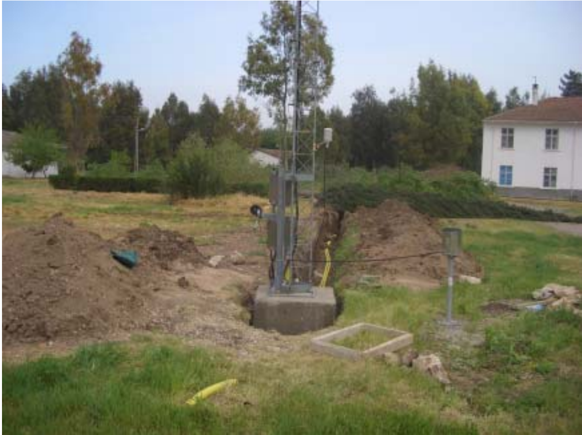
Picture 7: Cabling way is also important thing while selecting the place for AWOS
