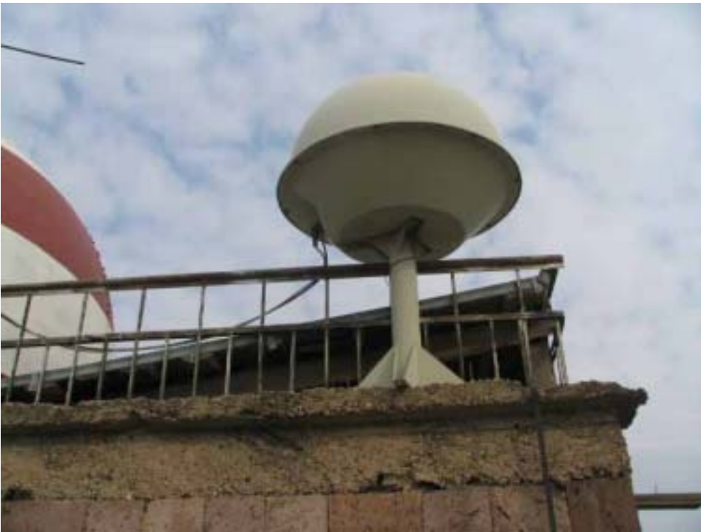
Figure 7, the stand was reused to mount the RB21 antenna.
