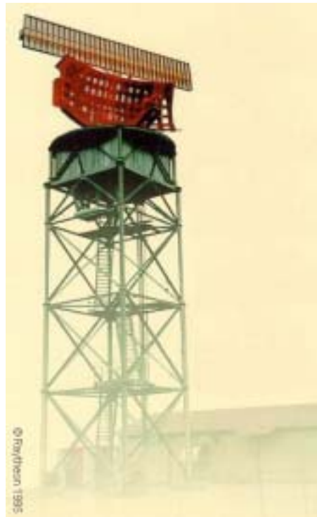
Figure 24: Air Surveillance Radars.
