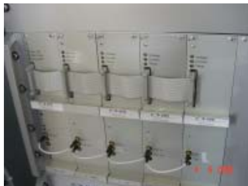
Figure 32: Modulator of a Transmitter.
