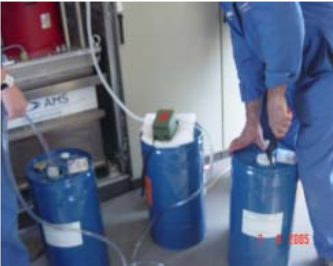
Changing Klystron Tank Oil
