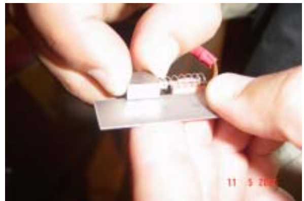
After Cleaning of the Slipring, The Length of Brushes Must Be Checked.
