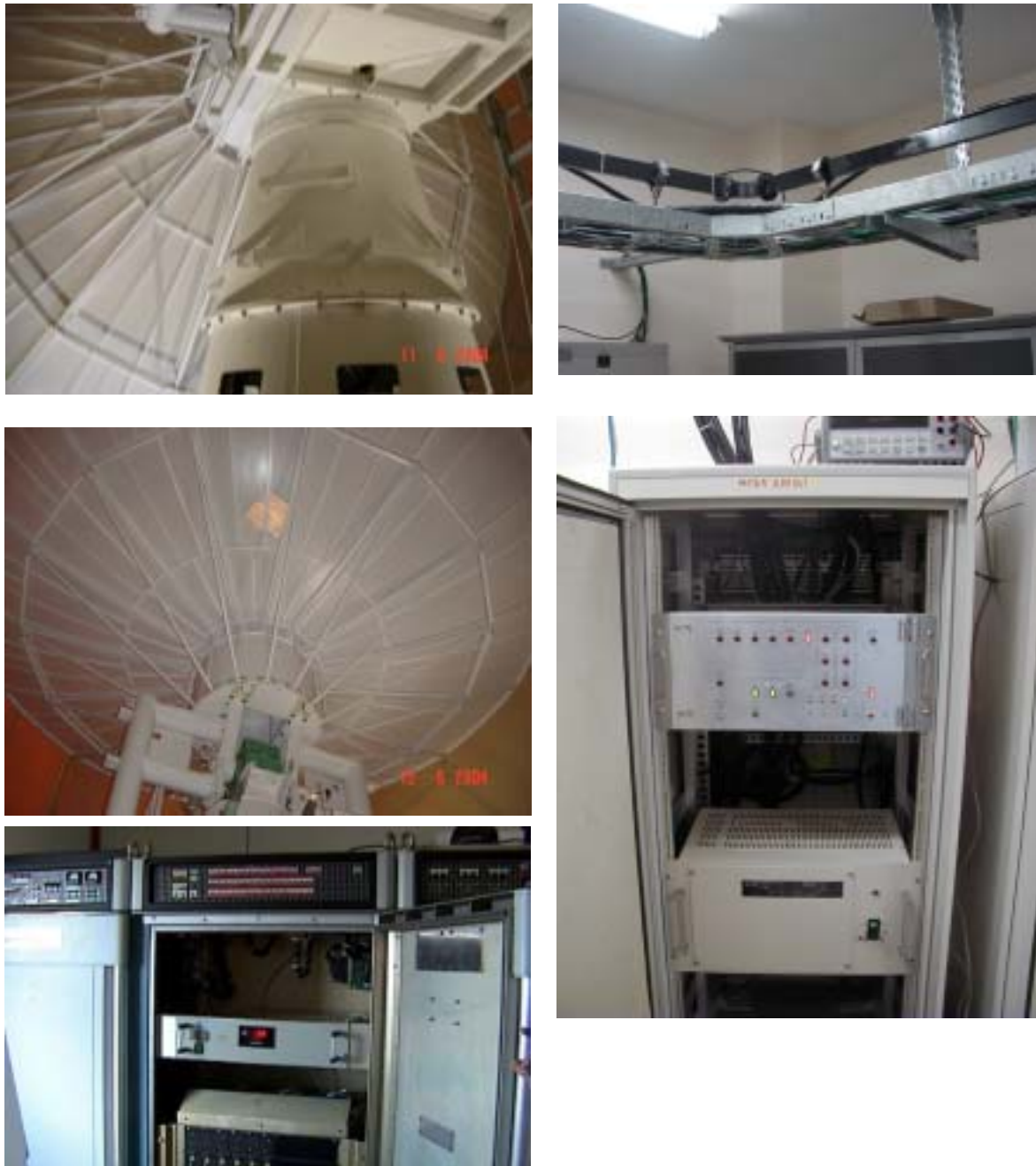
Figure 52: Some Pictures on Dehydrator, TX Cabinet, Cable, Waveguide and its Tray, 7m Parabolic Antenna, Antenna Pedestal, Obstruction Lights, Position Resolver of Antenna, Antenna Control Unit and Servo Amp., Antenna Control PCBs, Servo Amp., Angle Detector, Controller, Servo Motor.
