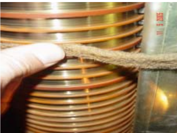
Cleaning of Slipring by Using Hard Sponge.
