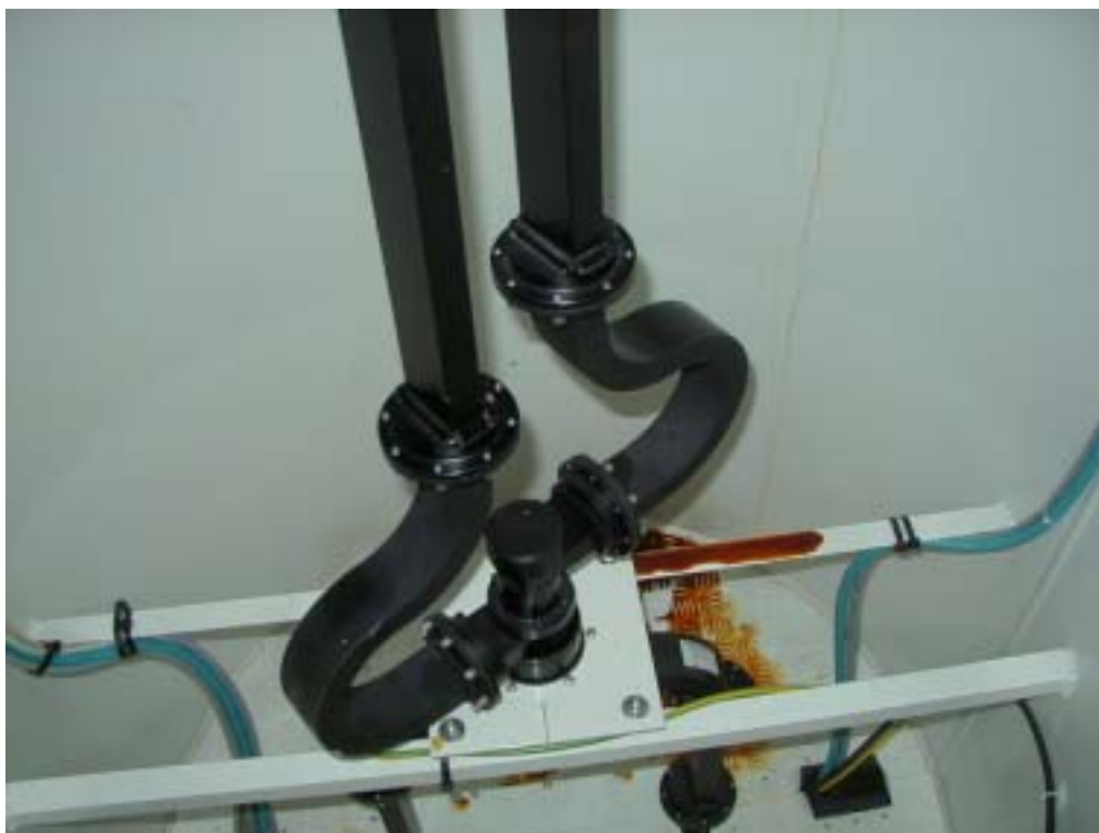
Figure 44: Rotary Joint.
