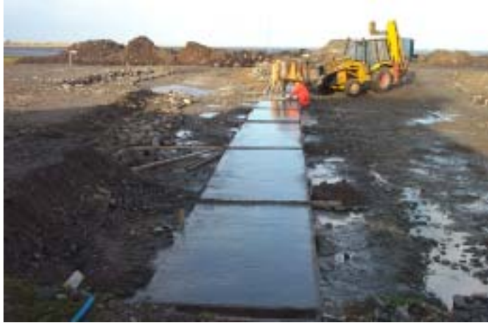
Figure 3 – Start of site preparation.
