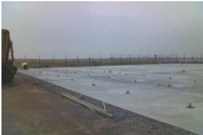
Figure 5 – YAGI Mountings.
