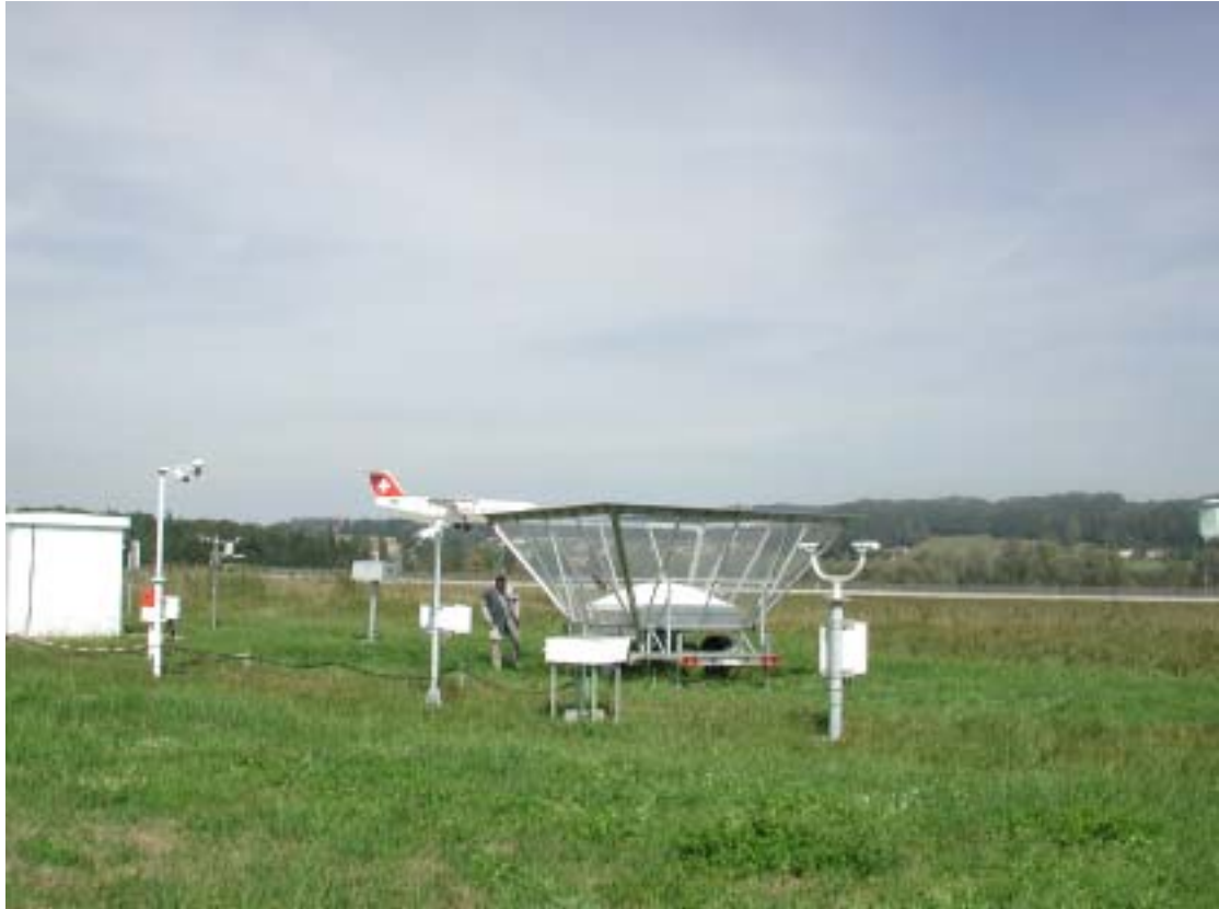
Fig.5(a) Temporary installation of Meteo Suisse-DWD wind profiler at Zurich airport.
