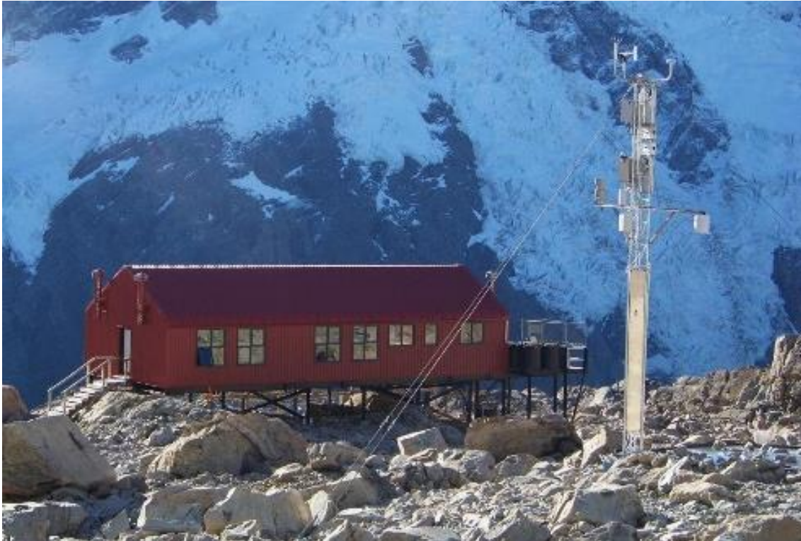
Figure 4: The Mueller Hut EWS as originally set up, with the Hut in the background. The snow pillow is visible at the base of the mast under the ultrasonic snow depth sensor.
