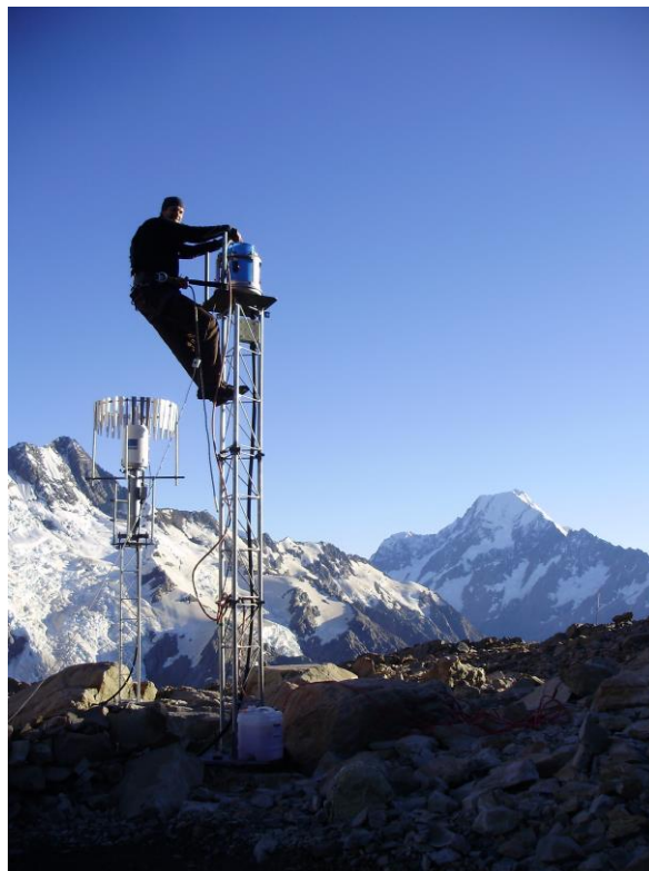
Figure 10: Technician putting in antifreeze mix on G2. With no snow cover, height access and work positioning equipment must be used.
