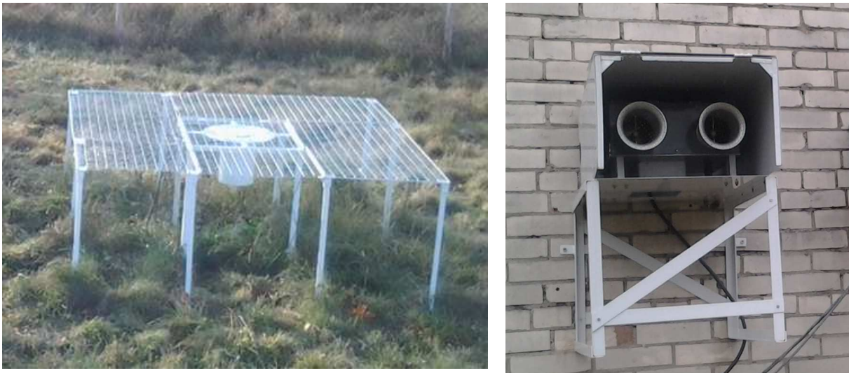
Figure 3. The ground-based sensors installation example.
