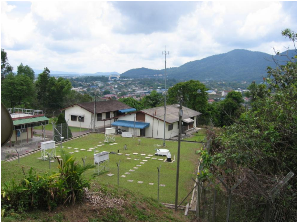
Automatic Weather Station (First Phase)
