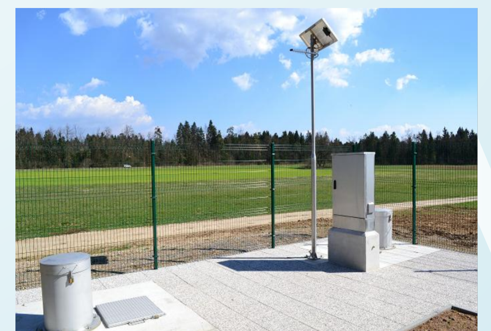
Figure 6: Photo of low power ground water X-DEG based station at location Meja Slovenia
