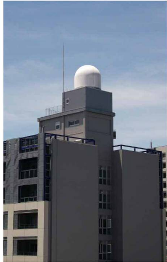
PAWR installed in Osaka Univ.
