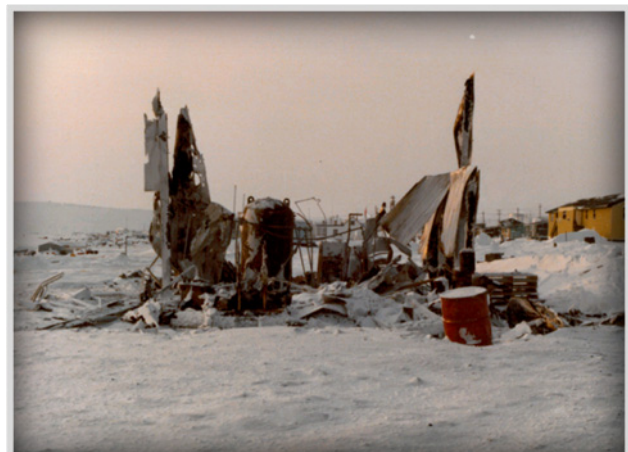
Figure 4.2: The aftermath of a hydrogen incident in Baker Lake, Nunavut -1979. No injuries occurred however the building was destroyed.
