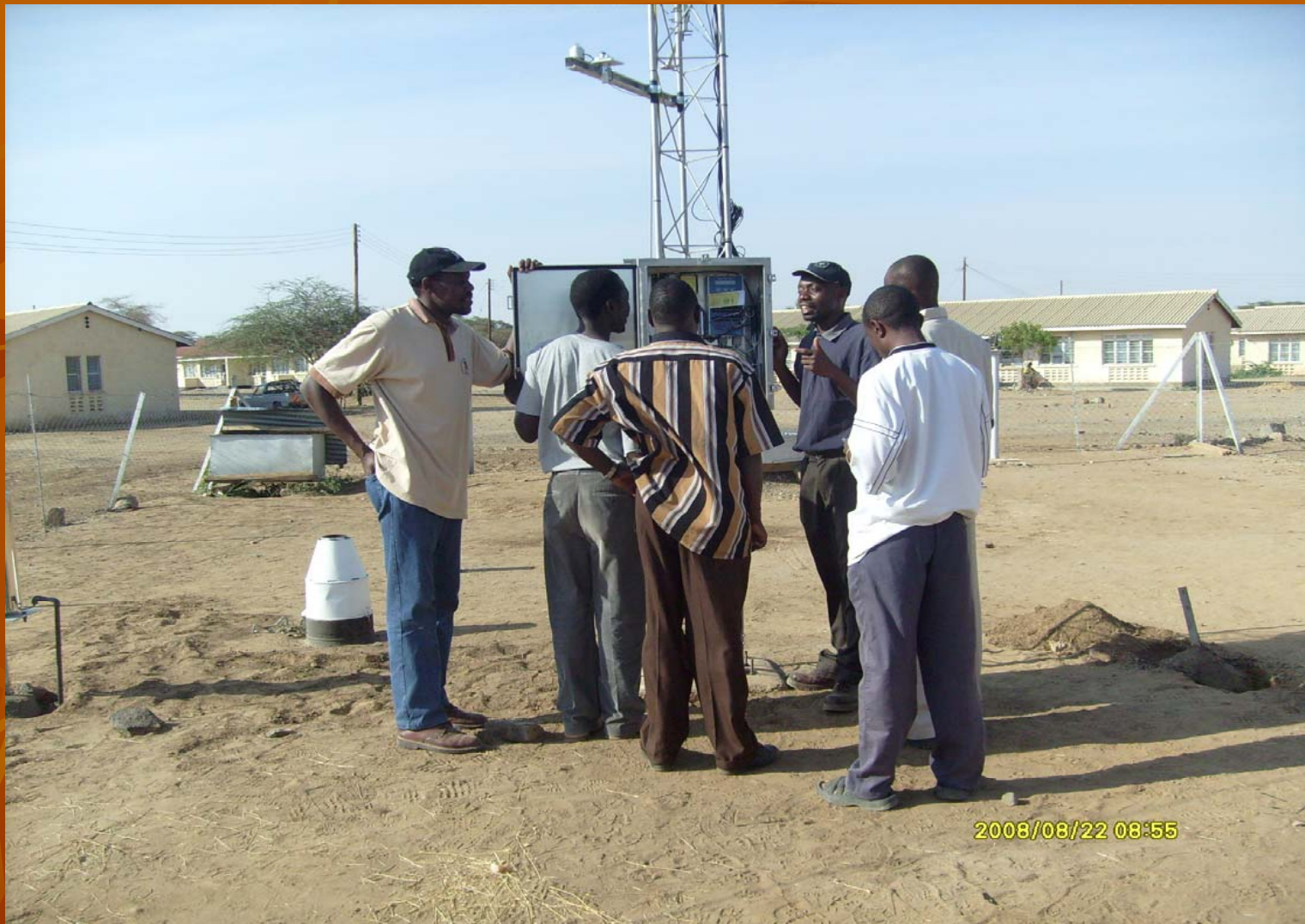
AWS INSTALLATION AT LODWAR- Figure 6
