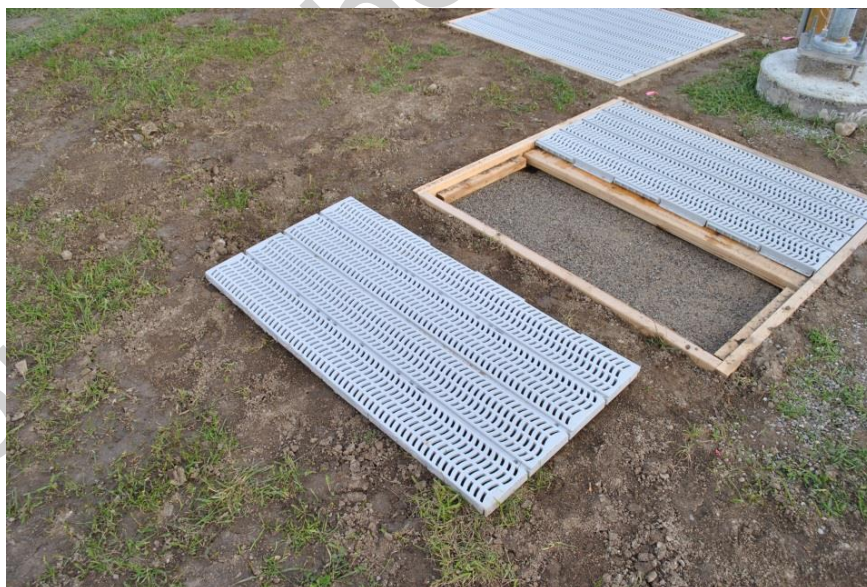
Figure 2.10. Perforated and textured grey plastic target during construction, with dimensions of approximately 1.2 m x 1.2 m installed on a constructed frame. (Photo courtesy of Environment and Climate Change Canada).
