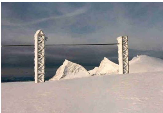
Figure A. 6 Norwegian rack for measuring ice loadings in remote areas
