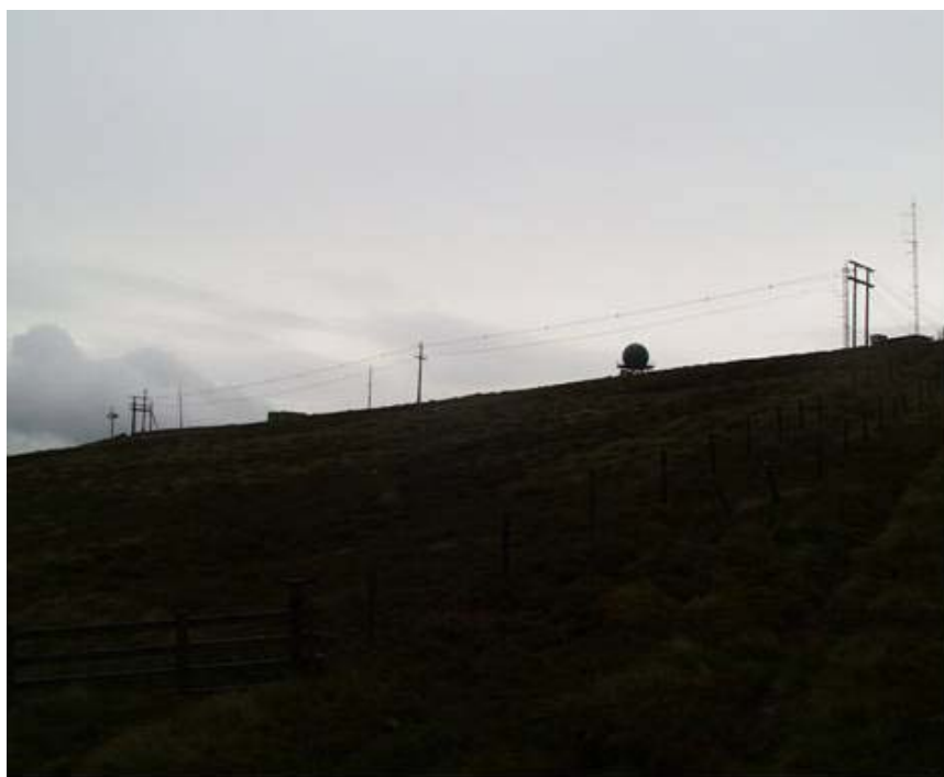
Figure A. 13 The full 200m span at Deadwater Fell
