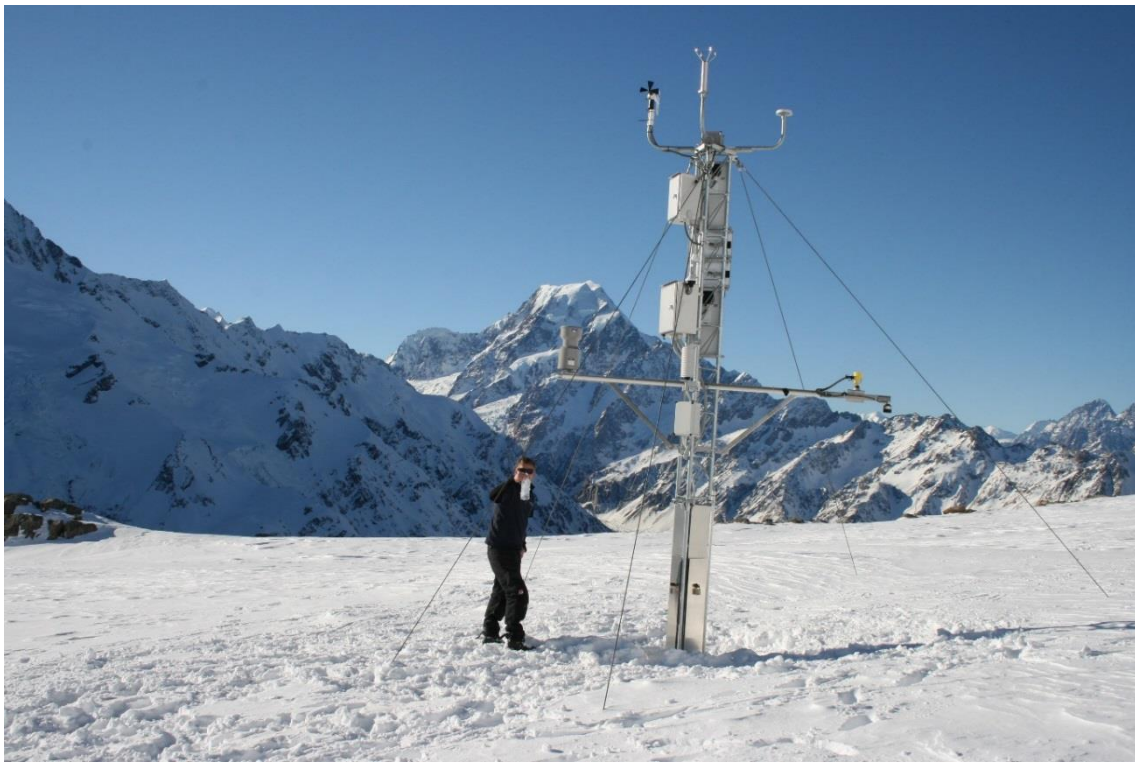
Photo 13: General mast layout (Vega radar and Vaisala wind sensor no longer present – December 2012). SR50A located on the right-hand protruding arm.
