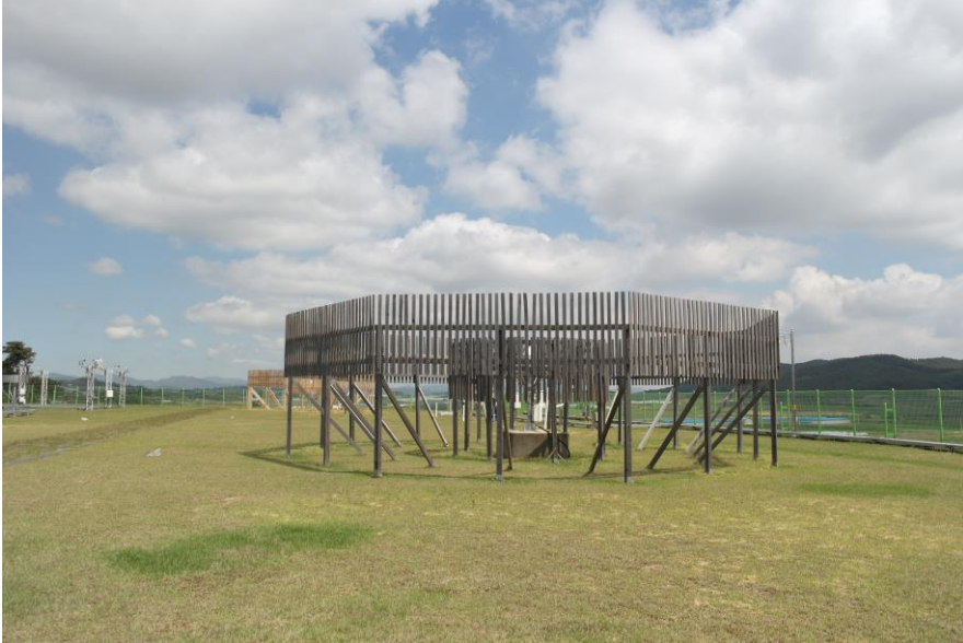
Photo of installation – DFIR (South)
