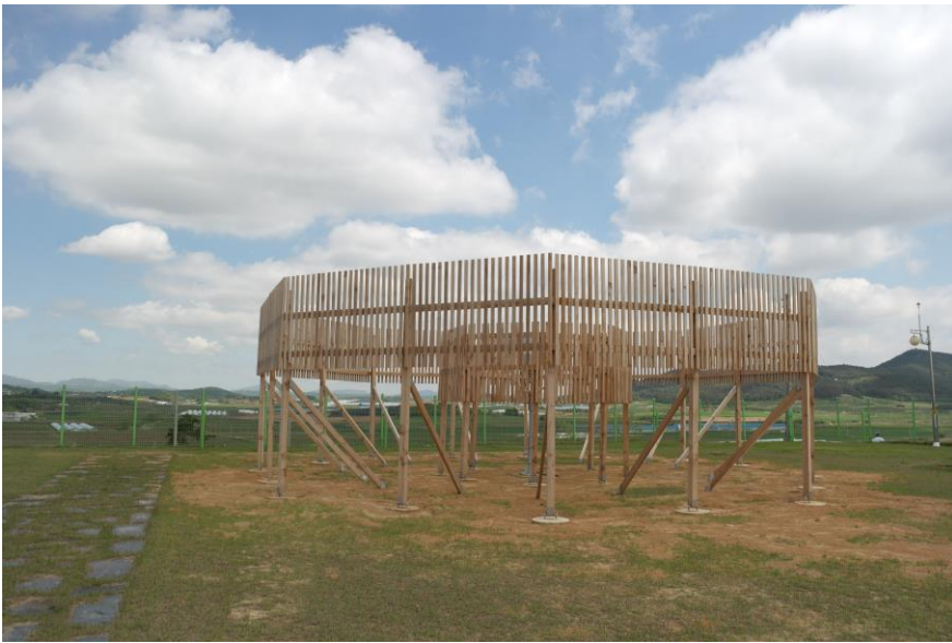
Photo of installation - DFIR (North)
