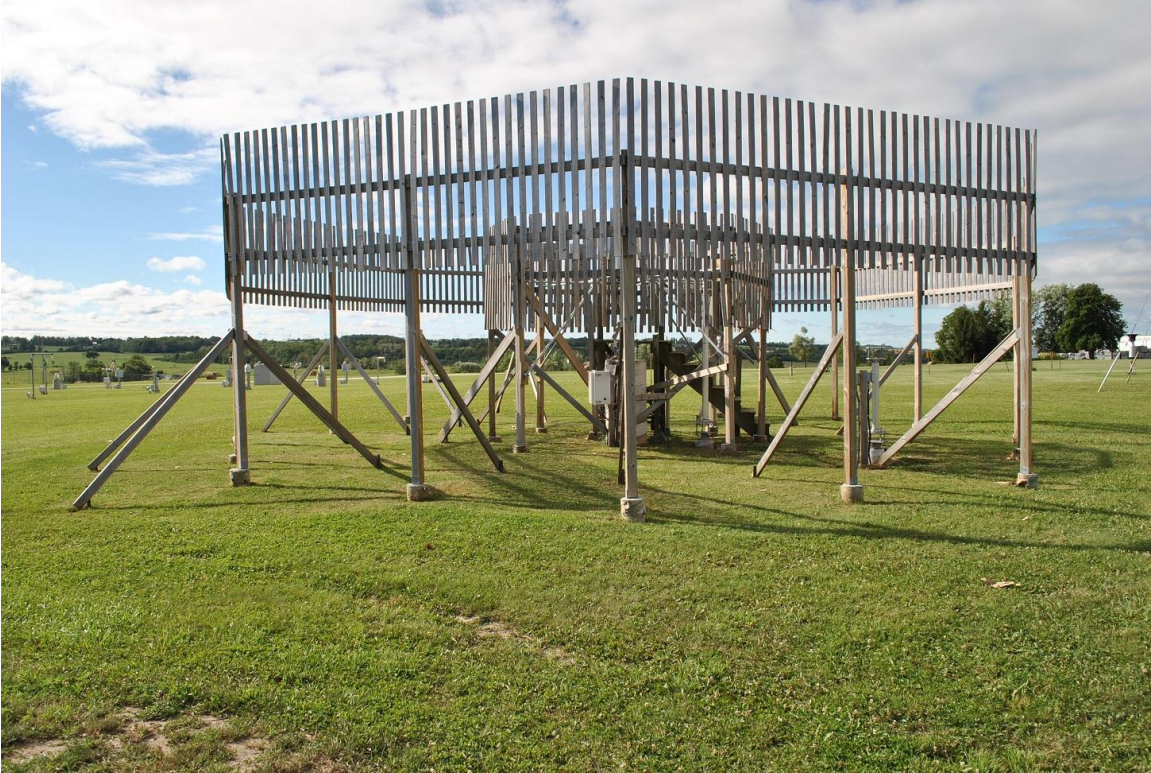
Photo of installation - DFIR shield
