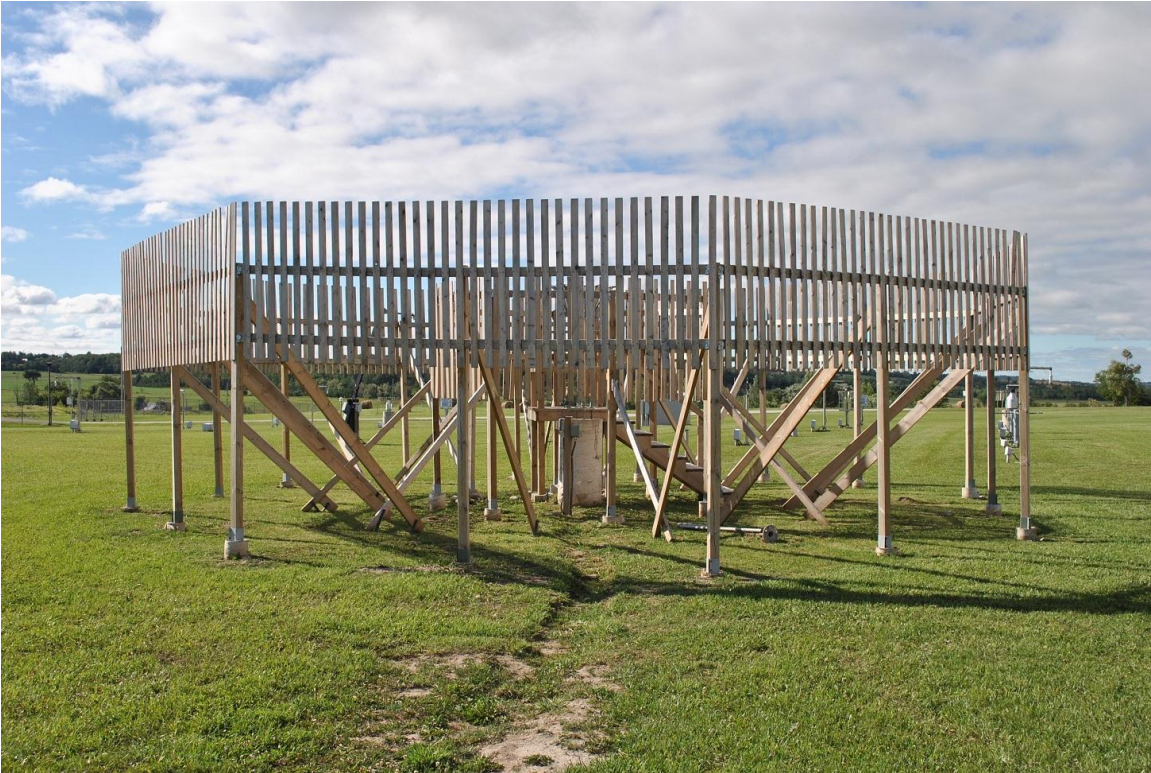
Photo of installation - DFIR shield
