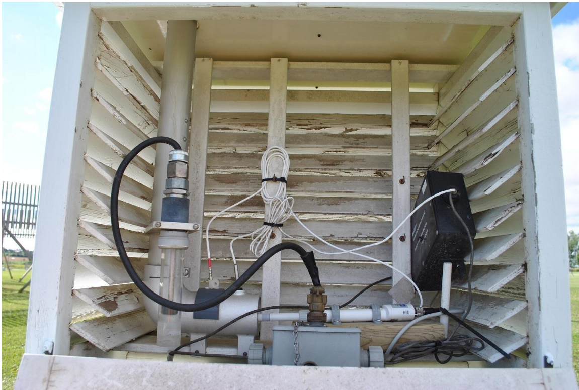
Photo of installation - inside Stevenson screen
