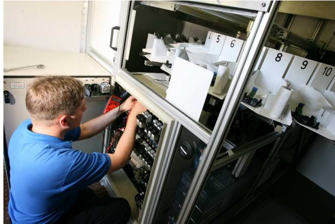
Figure 6. Corrective maintenance in progress at an automatic sounding station.
