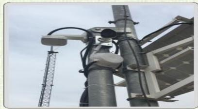
With cameras and motion sensors installed in station field, photographs of breach caused by human or animal movement are being uploaded to a server and audible alert is being created in the field.
