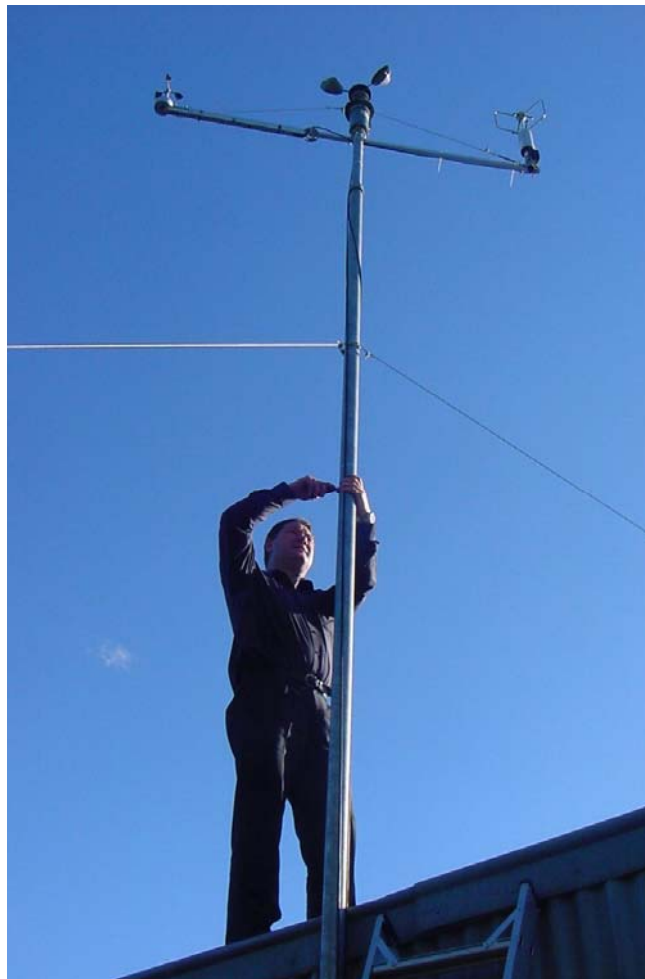
Figure 1. Collocated instruments and mast. The ultrasonic is at the right hand end of the cross arm, the Synchronotac in the centre and a Vaisala WAA151 on the left end.
