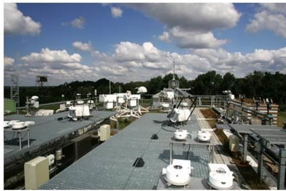
The roof platform of the radiation laboratory building
