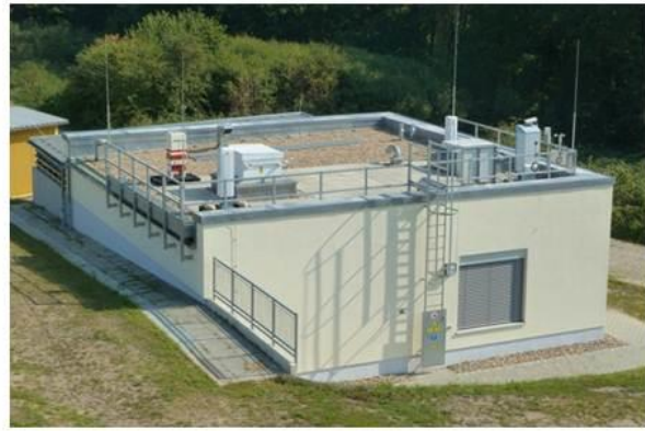
The lidar laboratory building with the roof platform
