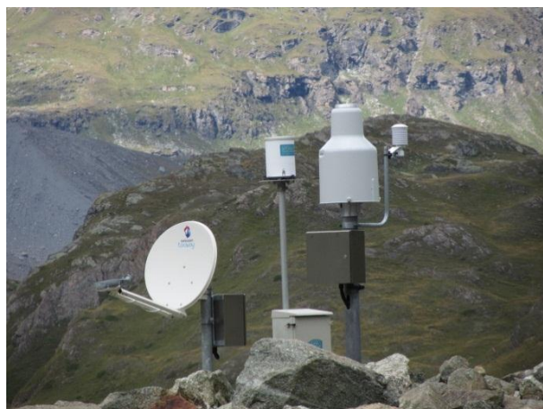
Figure 11. SwissMetNet automatic precipitation station with data transfer via satellite.
