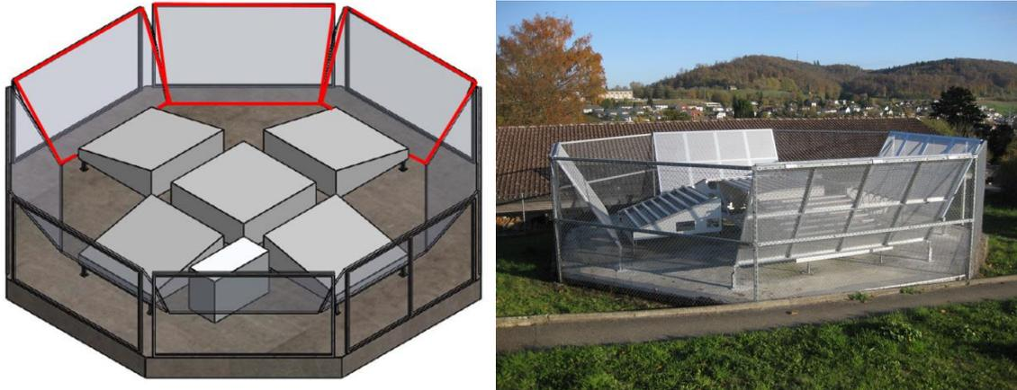
Figure 6: Design (left) and realization (right) of the new additional clutter fence panels. Based on cost-benefit considerations, only 4 out of 8 panels have been installed..
