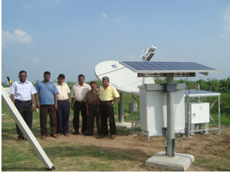
Fig. 3 Solar panels of AWS
