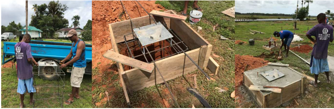
Figure 3 Construction of the AWS foundation at Santa Rosa, Guyana
