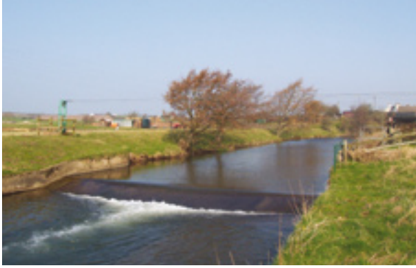
Figure I.7.14. River Ellen at Bullgill. North West England: Flat-v low flow control weir.
