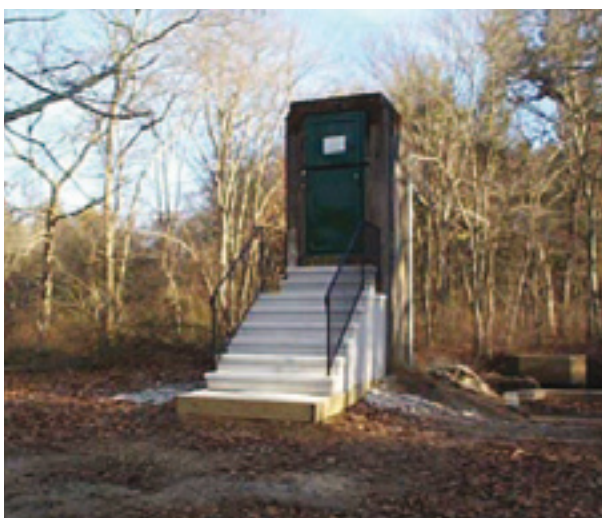
Figure I.4.1. Reinforced concrete stilling well and shelter
