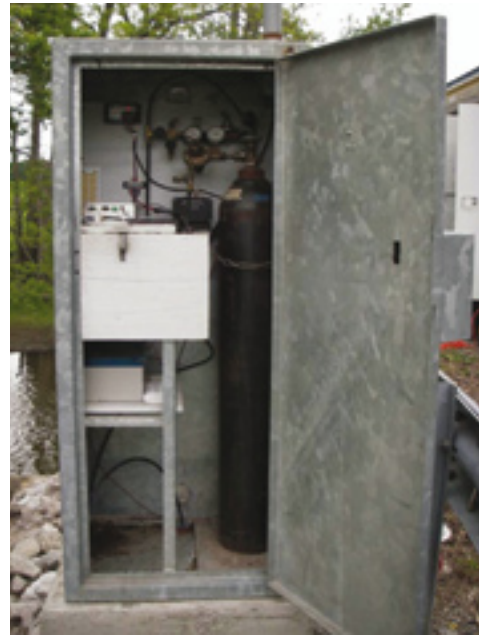
Figure I.4.9. Instrument shelter located on a stream bank
