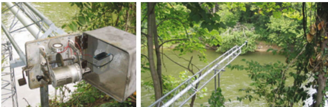
Figure I.4.18. Horizontally cantilevered wire-weight gauge
