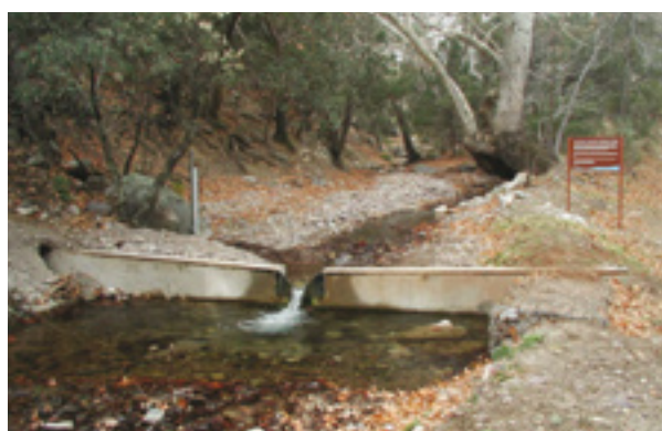
Figure I.3.5. A concrete, broad-crested artificial control with a shallow V notch in the centre
