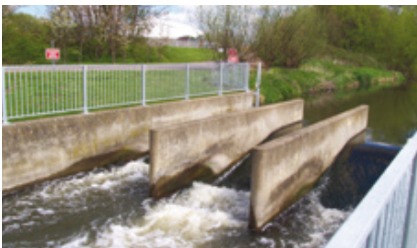
Figure I.7.15. River Colne at Berrygrove. South East England. Compound crump weir.
