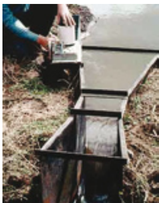
Figure I.3.3. A Parshall measuring flume
