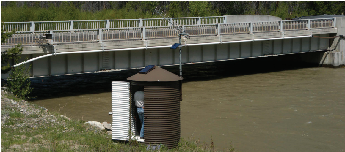
Figure I.2.1. Gauge with walkin shelter, solar panels, satellite antenna, and wire-weight gauge on bridge
