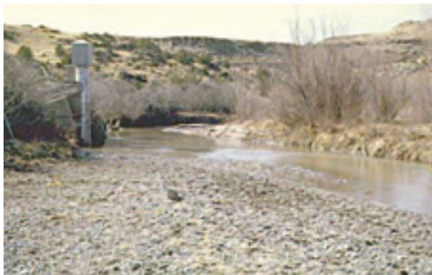
Figure I.3.1. Gauging stations with natural section controls
