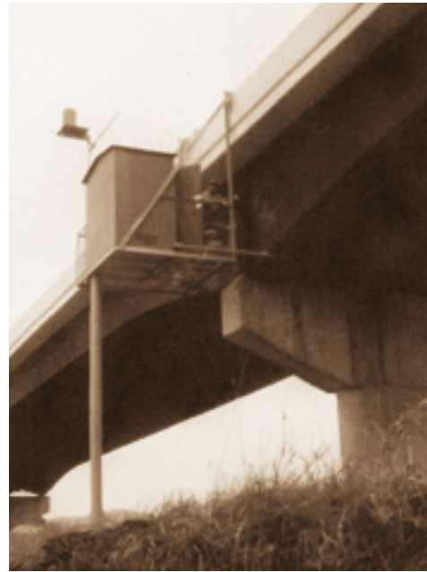
Figure I.4.10. Instrument shelter located on a bridge pier
