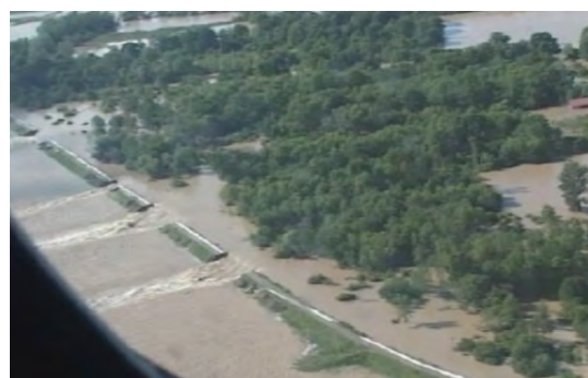
Figure 175. Embankments breaches in BiH
