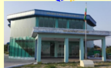
DMH Multi-Hazard Early Warning Center, Nay Pyi Taw
