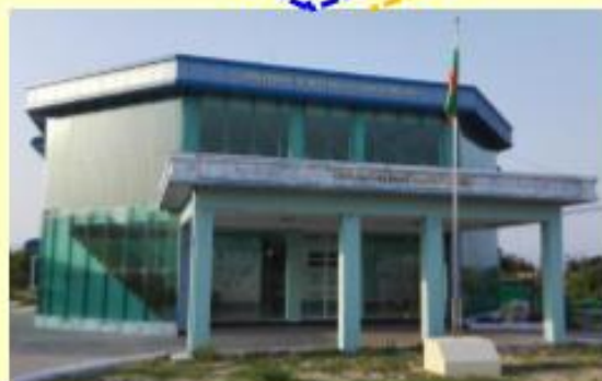
DMH Multi-Hazard Early Warning Center, Nay Pyi Taw
