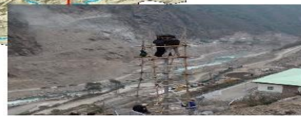
Punatshang Chhu I Power house Siren
