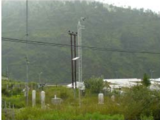
Photo 4: Automatic Weather Station installed at Semtokha, Thimphu along with rain gauge
