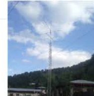
Control Center at Kurje Site Office
