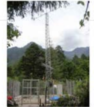
Automatic Water Level Station at Khagthang
