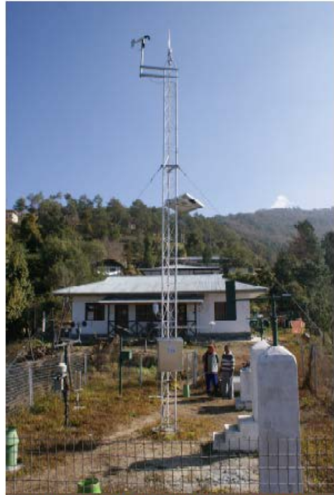
Photo 8: AWS installed at Kanglung, Trashigang
