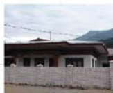
Mingkar Control Center
