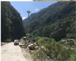
Siren at MHPA Dam Site
