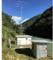
Automatic Water Level Station at Bjizam
