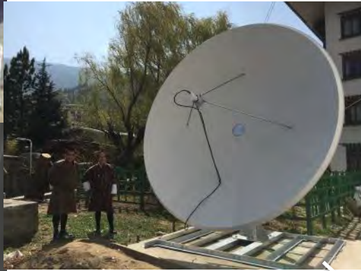
Satellite image receiver (HimawariCast)
