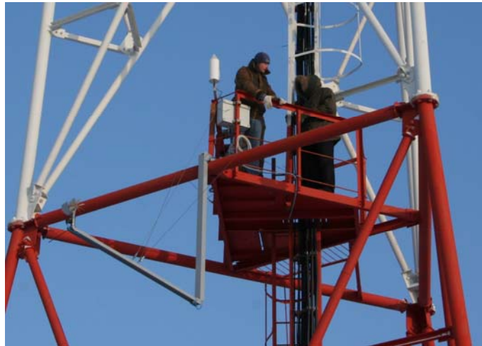
Installation of the communication kit
