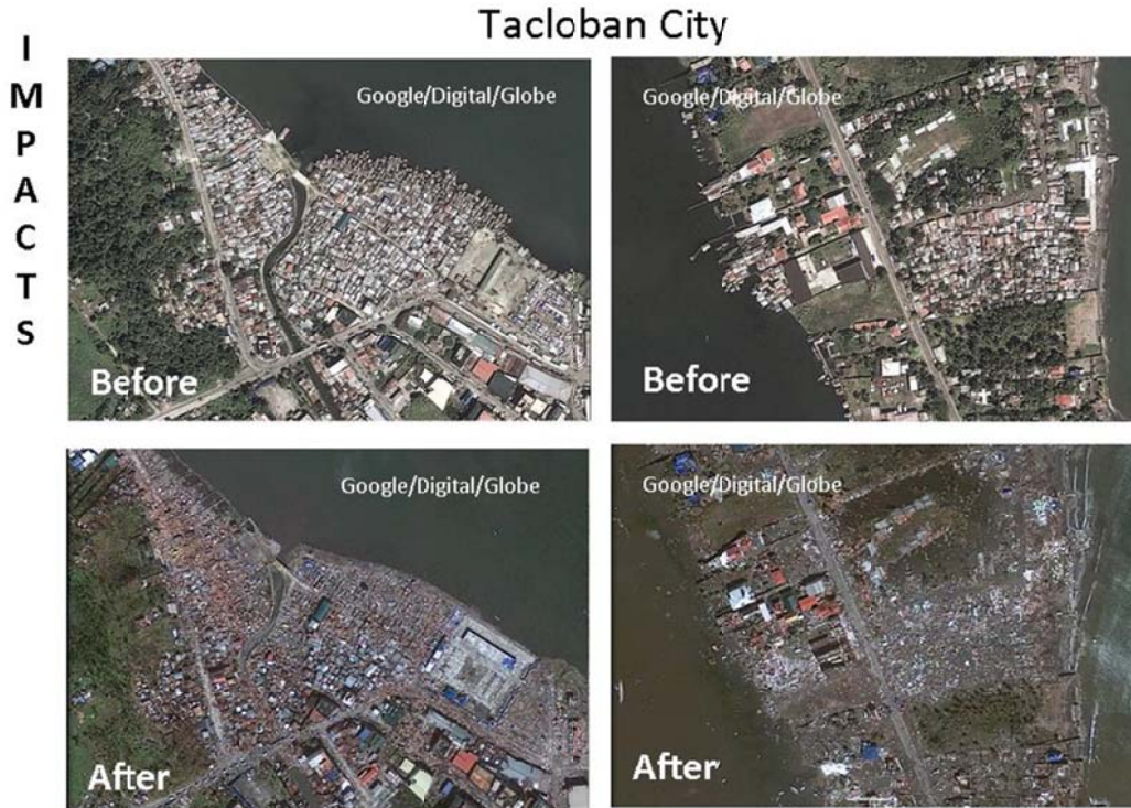
Fig. 5 - Damage caused by Haiyan in Tacloban City
