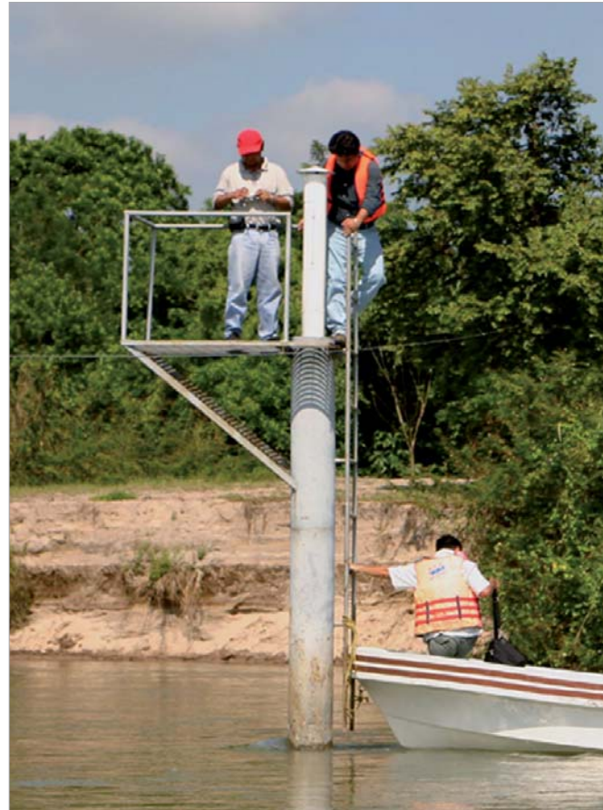
The Thalimedes sensors installed in river basins permit to measure the water level in an hourly basis (photo PROMMA).
