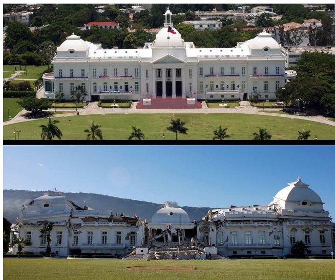
Haiti's National Palace before and after the earthquake
