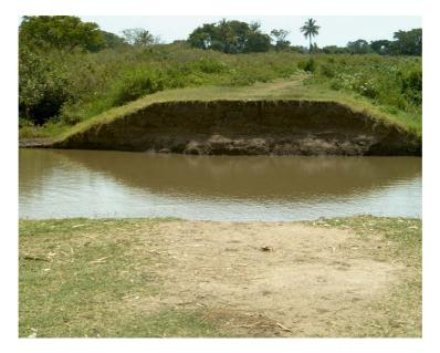
A broken dyke on the River Nzoia caused by the August 2003 floods in the Budalang'i area. The photograph was taken after flooding had subsided. (Photo courtesy of KMD)
