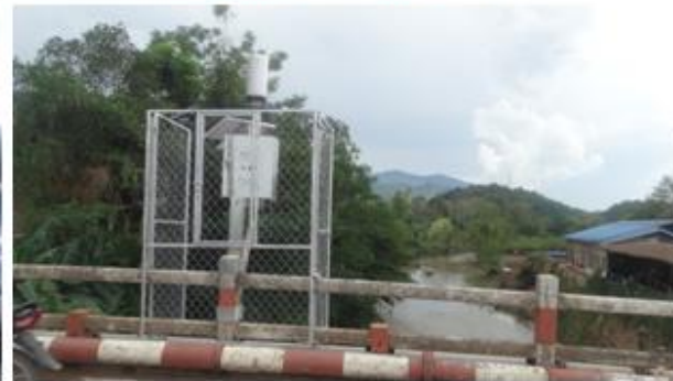
Nam Kor bridge 2
