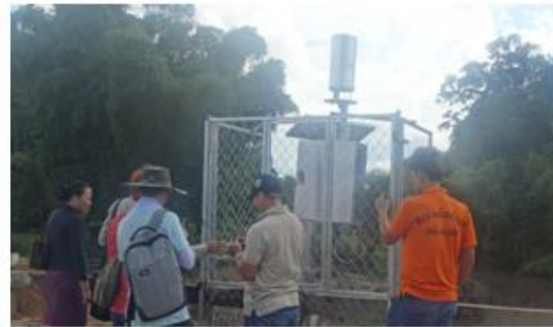
Ban Kor Noy , Nam Kor bridge 1
