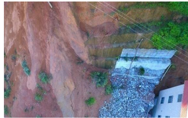
Aerial image of mountain cracks
