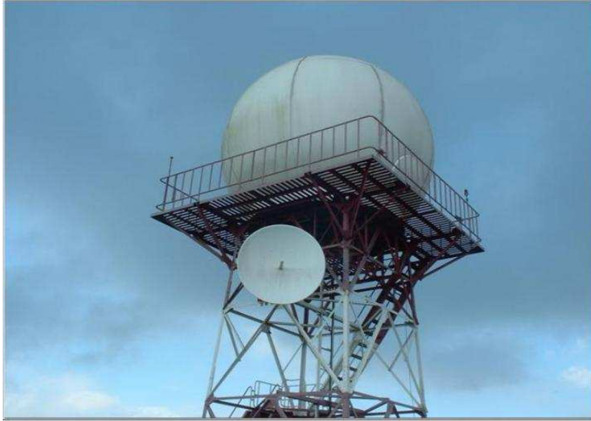
Plate 5a: Photograph of the Doppler Radar used for weather forecasting in Jamaica
