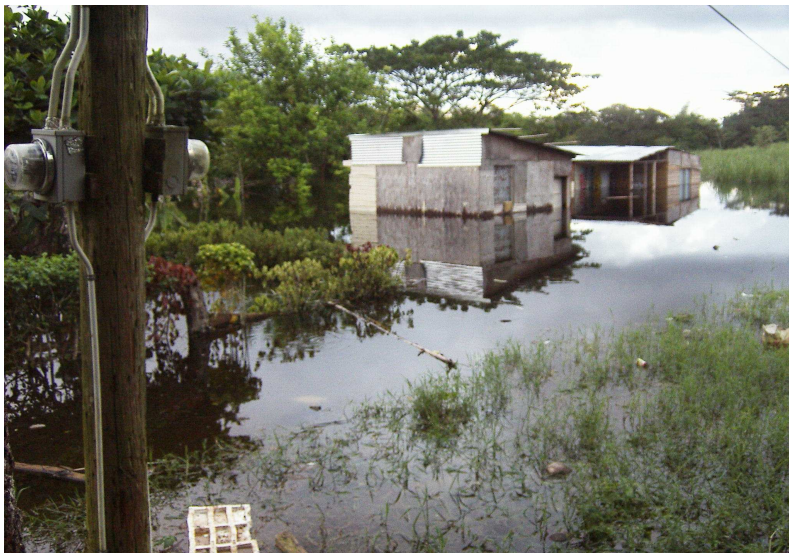
Plate 3b: Flooding of houses in a flood prone area in western Jamaica
