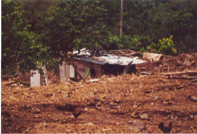
Plate 3a: Debris from flooded river partially destroyed a low-income dwelling
