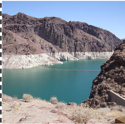
Runoff & flow into reservoir, water levels behind dam
