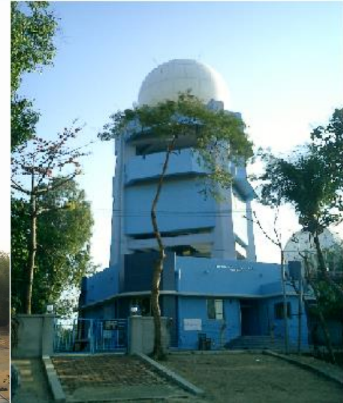
Cox's Bazar Radar
