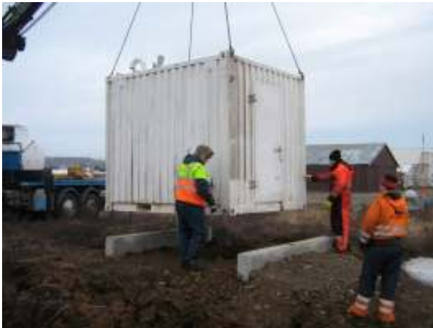
Installation of ASAP station at Egilsstadir Airport, Iceland
