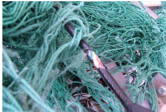
Figure 7. Modem Cable Damaged by Fish Net Entanglement - Indian Tsunami Buoy
