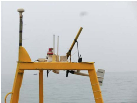
Figure 2 Ship collision damage
