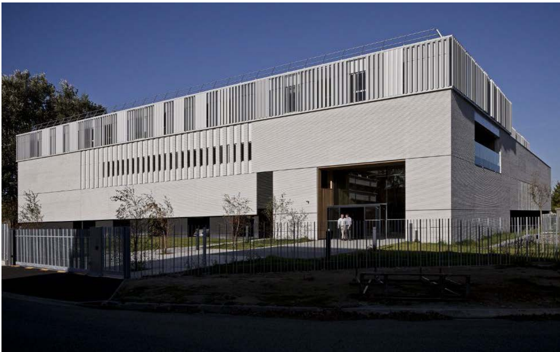
Figure 14 : CLS Toulouse new building
